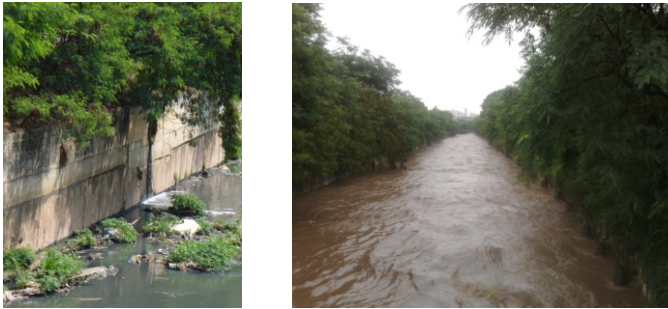
Figure 16. Sewage, garbage discharge and the flooding occurrence at Pirajuçara River - Metropolitan Area of São Paulo.
